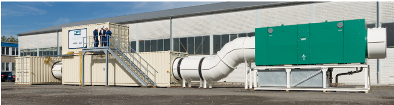
Fig. 5: Assembly of the ventilation system for number 2 shaft at the factory
