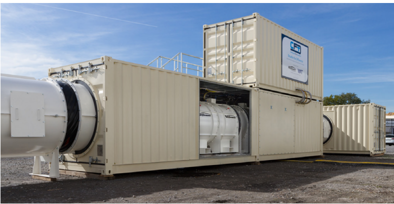
Fig. 6: Service hatch (shown open) for fan container with axial fans behind
