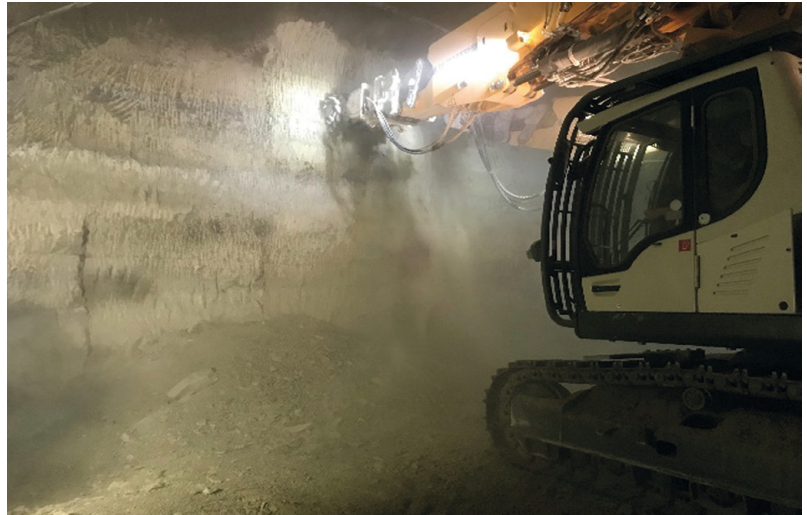
Fig. 1: Tunnelling with a cutter-head excavator
