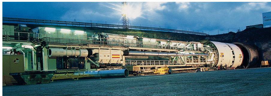
Fig. 3: Full-face mechanised heading
