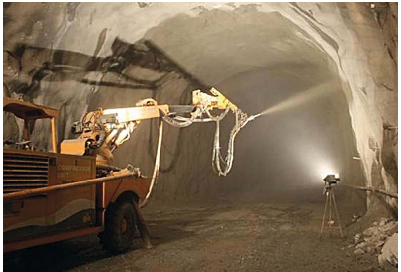
Fig. 2: Shotcreting in a tunnel drive
