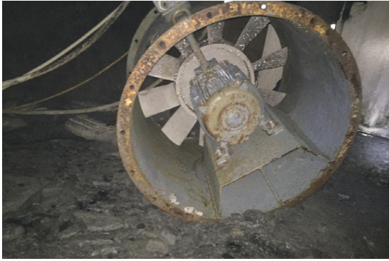
Fig. 3: Handling below ground
