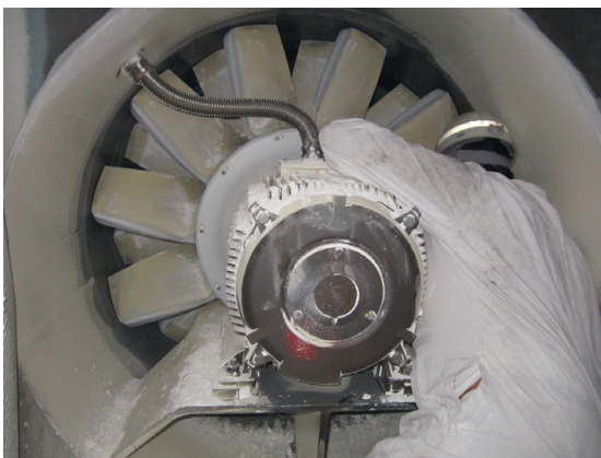
Fig. 10: Fan affected by airborne salt particles
